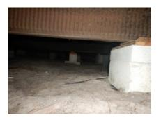
**1.19 Piers Rest On**Masonary block and ABS pier base
